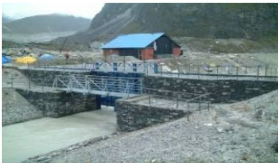
Figure 32. Outlet channel constructed to facilitate the lowering of Tsho Rolpa, Nepal. Image from CEPAD Hydro Consultants 433 .
