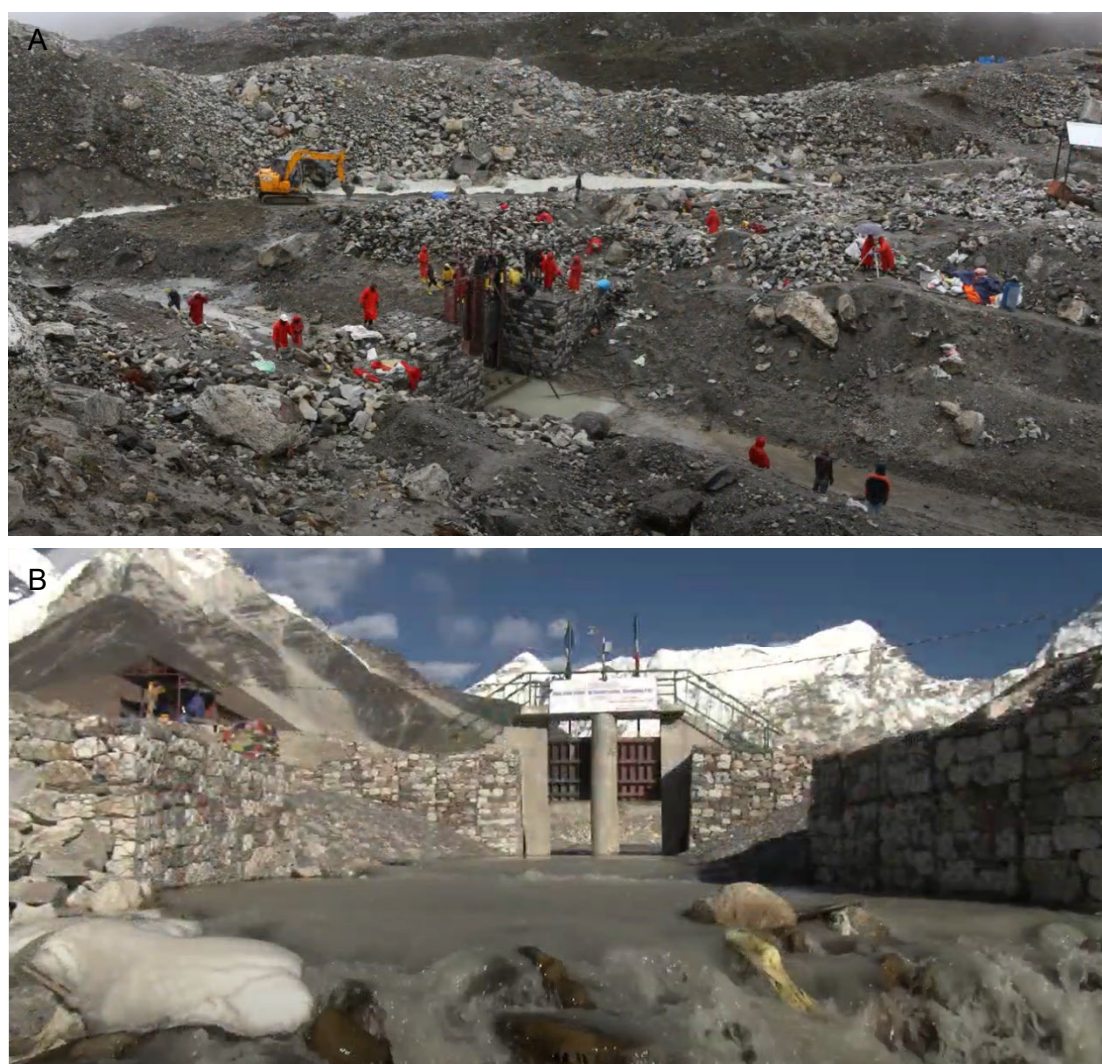
Figure 35. The excavated outlet channel of Lake Imja under construction (A) and complete (B) 442 .
