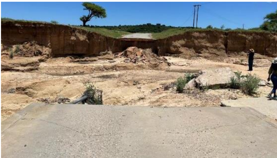
Figure 4-26: Bridge washed away near Kraai Pan during flooding, Ngaka Modiri Molema DM
