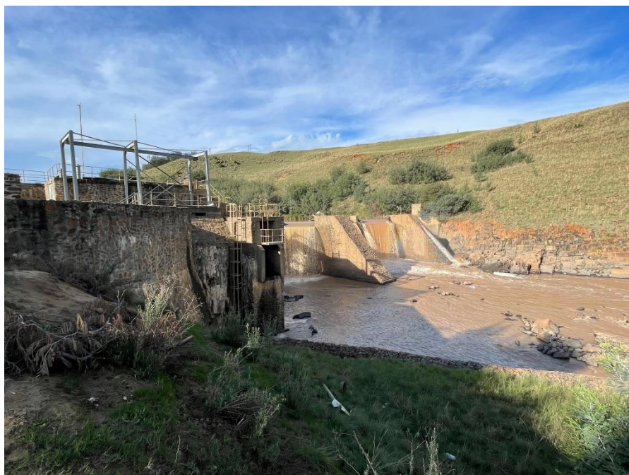
Figure 4-21: A dam in Joe Gqabi DM that has reduced capacity due to siltation
