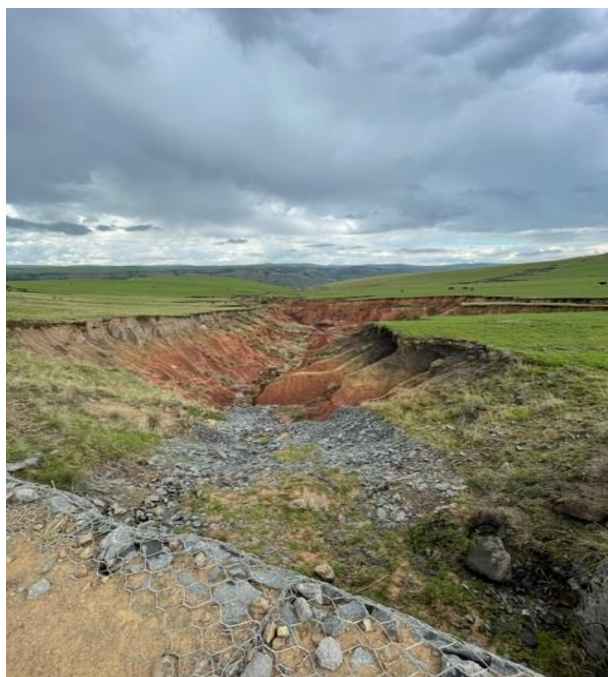
Figure 4-24: Donga erosion below road culverts
