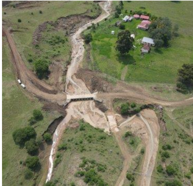
Figure 4-17: Example of erosion and flood extent threatening a bridge in Alfred Nzo DM
