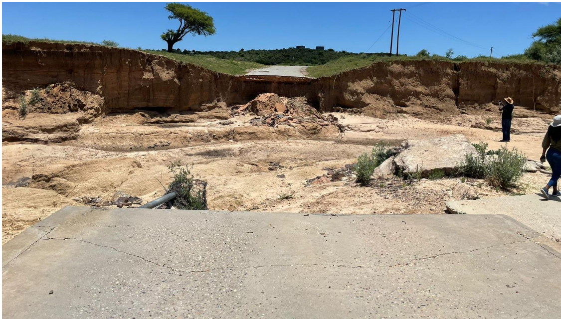
Figure 4-70: Bridge washed away in Kraaipan during flooding, Ngaka Modiri Molema DM
