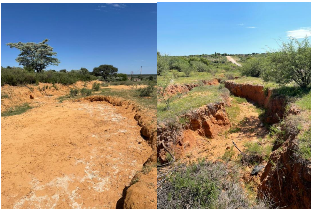
Figure 4-71: Donga development alongside roads in Ratlou LM that experience flash flooding during extreme rain events
