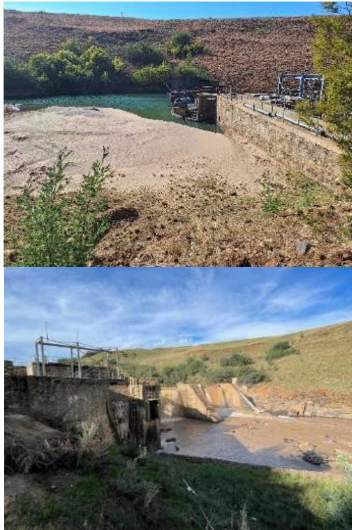
Figure 4-19: A dam in Joe Gqabi DM that has reduced capacity due to siltation
