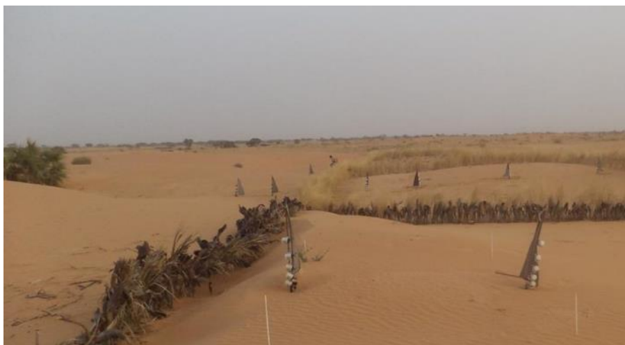
Figure 98. Check dunes have been successfully erected within the proposed project's target region to prevent the advancement of sand 891 .
