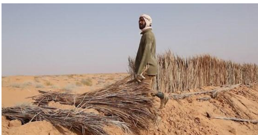
Figure 101. Wattling ( clayonnage ) constructed using bundles of dead date palm fronds 894 .
