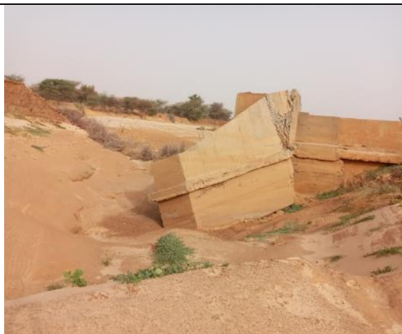
Figure 19. Examples of damage to infrastructure from flooding within the target hubs, including: i) ravine formation from erosion and road damage from runoff along the Taoujeft bridge near Rachid (left); and ii) damage to an embankment junction in Tamcheket (right).
