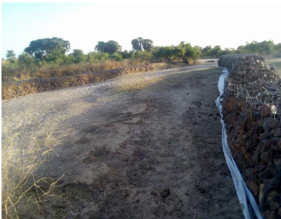
Figure 112. Stone gabion constructed in parallel with a watercourse within the proposed project's target region 980 .
