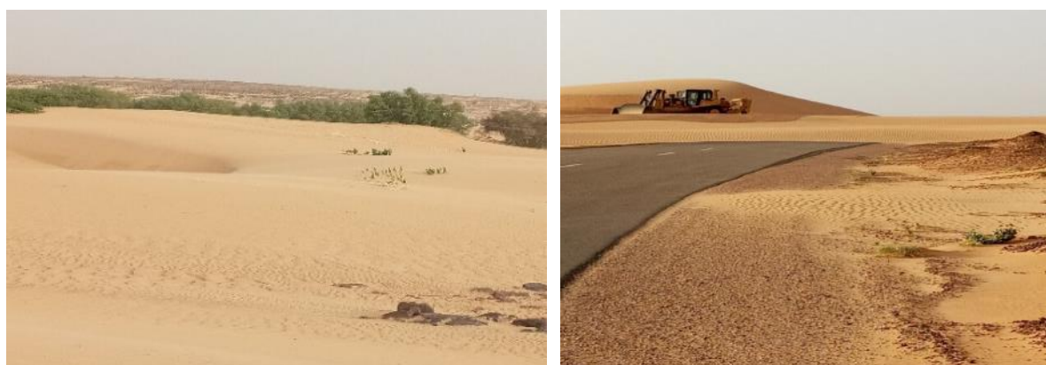
Figure 14. Examples of sand inundation from SDS and desertification, including: i) sand encroachment of an oasis in the Aoujeft hub (left); and ii) dune obstruction of a road (right) 321 .
