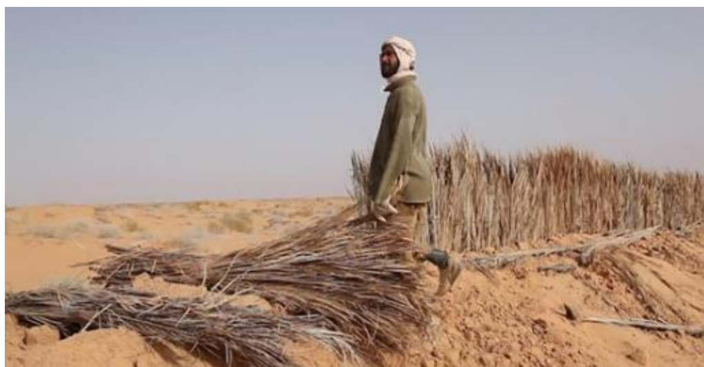
Figure 144. Wattling ( clayonnage ) constructed using bundles of dead date palm fronds 1076 .
