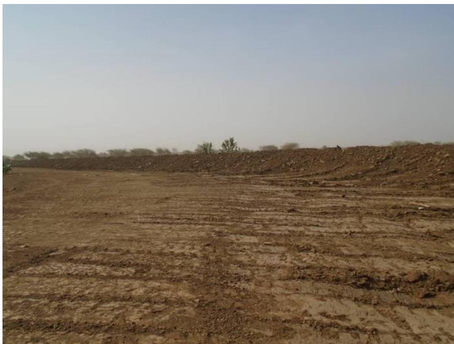
Figure 111. Clay dyke constructed within the proposed project's target region 979 .
