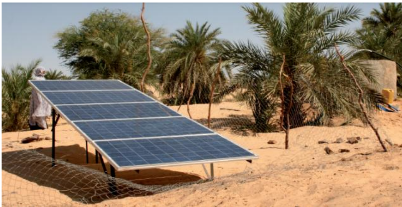
Figure 152. Solar-powered groundwater pump installed on an agricultural plot under the PDDO programme in Mauritania.
