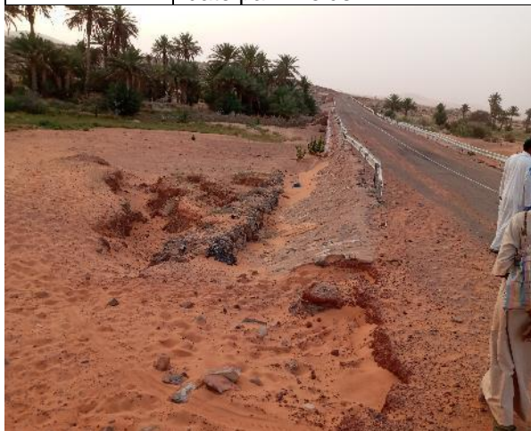
Figure 19. Examples of damage to infrastructure from flooding within the target hubs, including: i) ravine formation from erosion and road damage from runoff along the Taoujeft bridge near Rachid (left); and ii) damage to an embankment junction in Tamcheket (right).
