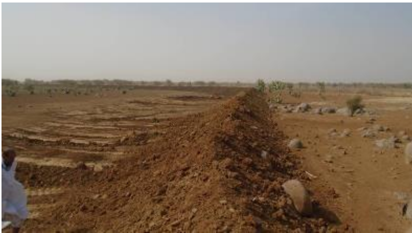
Figure 148. Clay dike constructed along a water course within the proposed project's target region 1098 .
