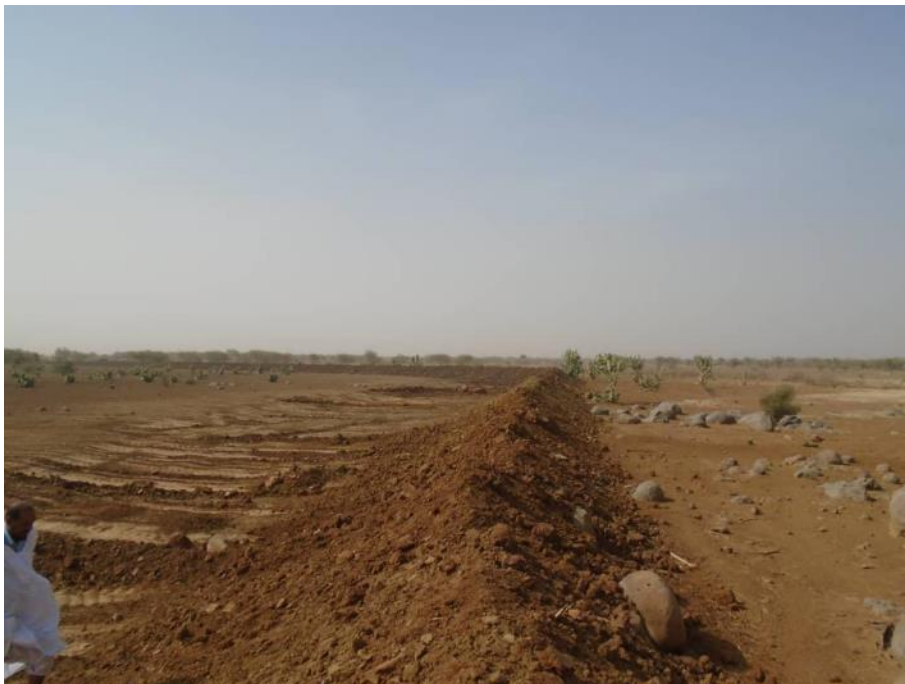
Figure 110. Clay dyke constructed along a water course within the proposed project's target region 978 .
