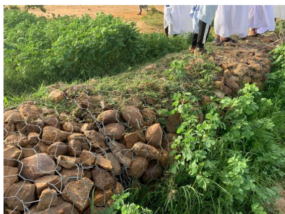
Figure 8: Bank stabilization (Ndoumally)
