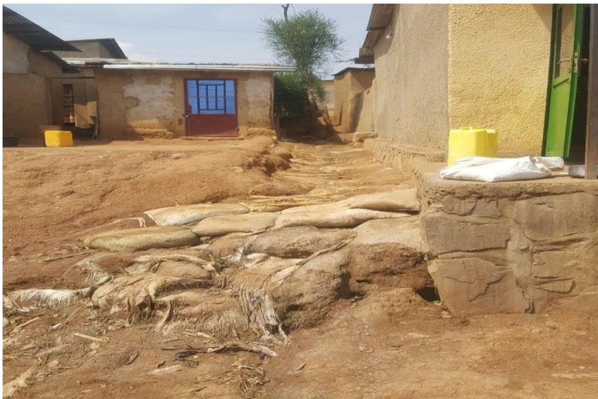
Figure 5-25 Poor storm water management infrastructure and erosion gullies sandbags
