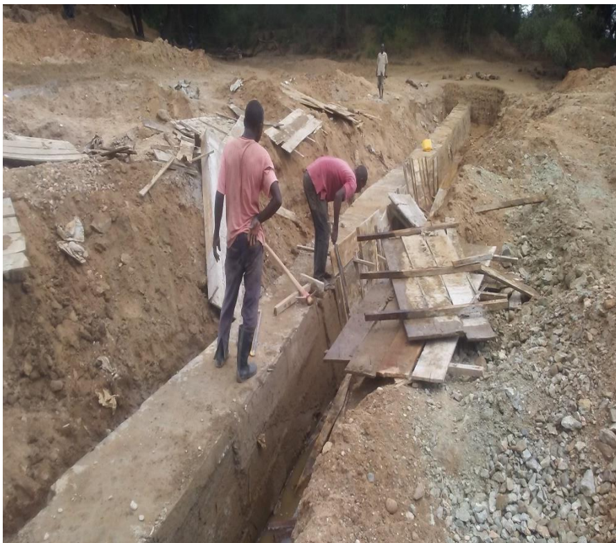
Figure 17: Lotiyan Subsurface dam under construction
