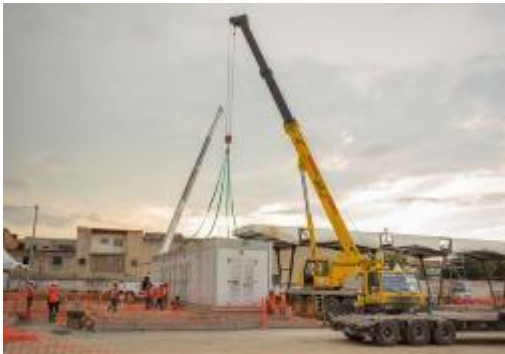
(a) Installation of mini substation in bus depot 49 (b) bus depot upgrade 50 (c) Bus charging station 51
