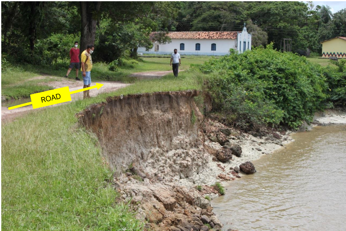
Figure 15. Bank landslide near the road in the Caldeirão community, Salvaterra/PA – 03/12/2022. Image: Wilson Cabral
