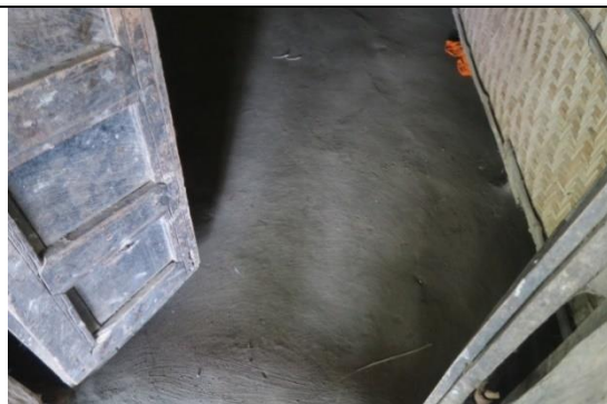
Figure 25: Indoor floor with mud
