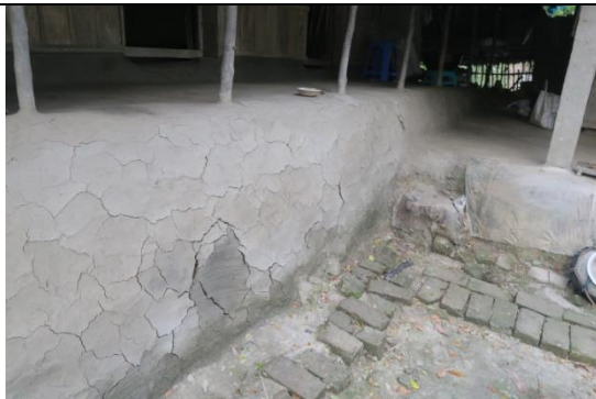
Figure 22: A meter height of plinth with cracks
