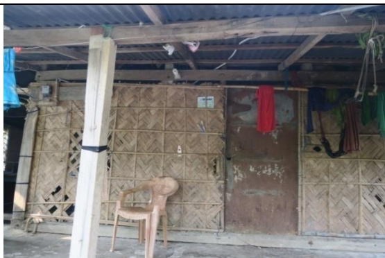
Figure 24: Bamboo wall structure
