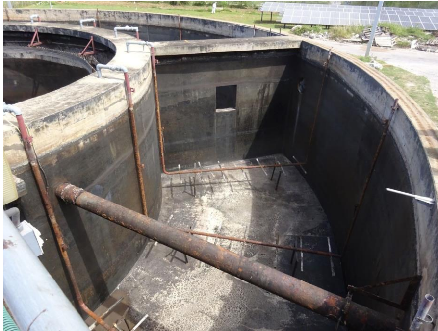
Figure EE. Contact Stabilization Bioreactor (Undergoing Replacement of Diffusers)
