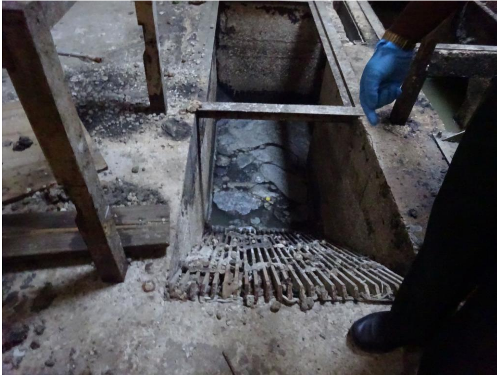
Figure CC. Inlet Trash Rack
