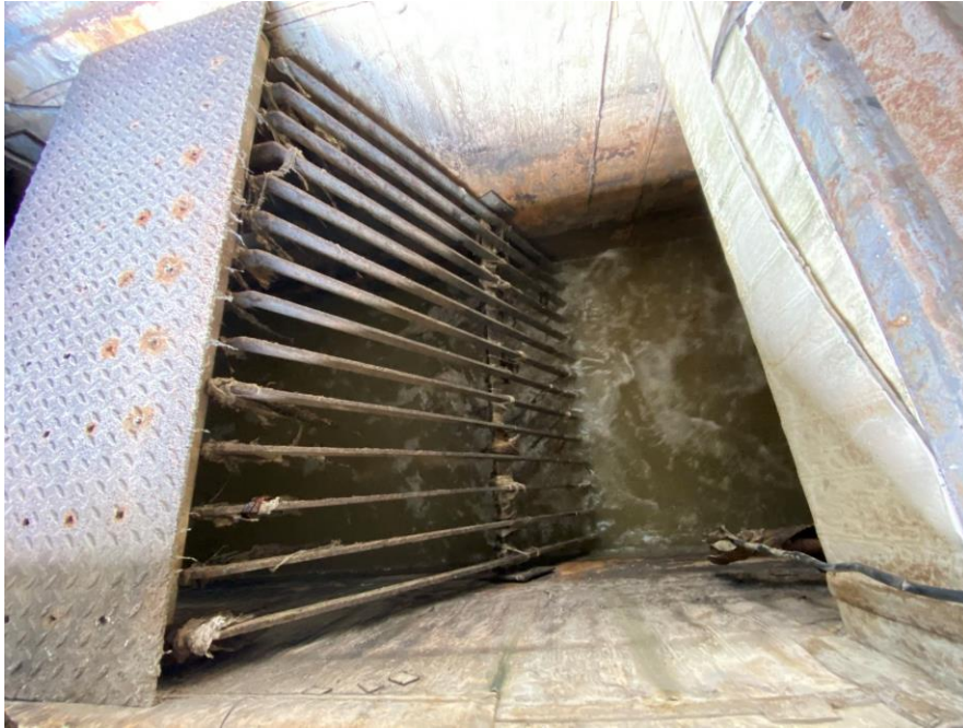
Figure U. Inlet Screen - Trash Rack
