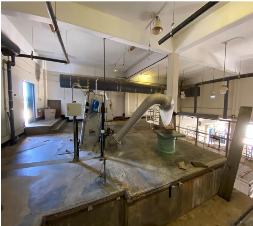
Figure V. New Coarse Screen System
