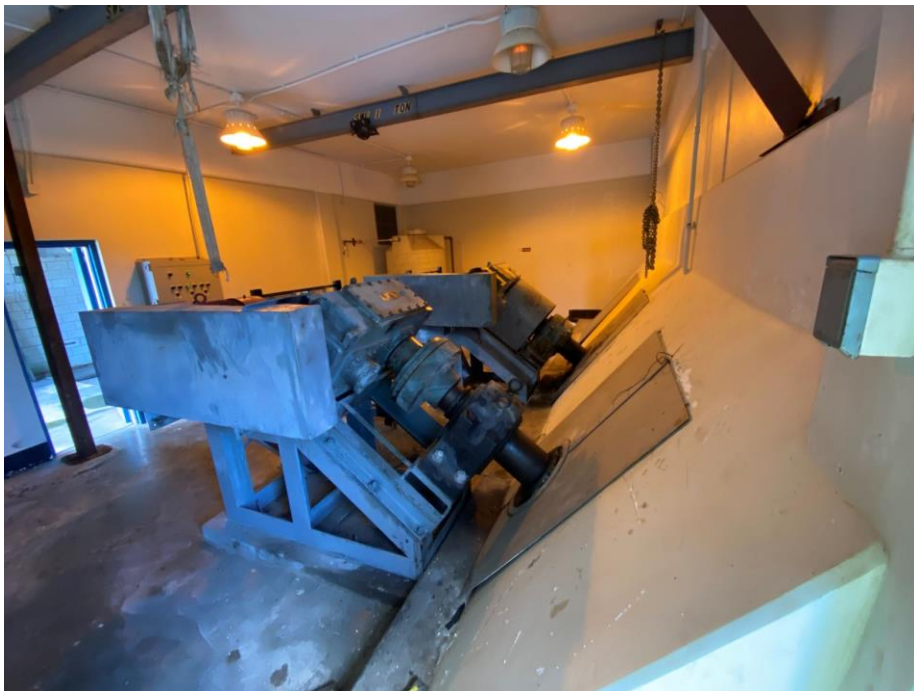
Figure T. Screw Pump System (Top of Channels)
