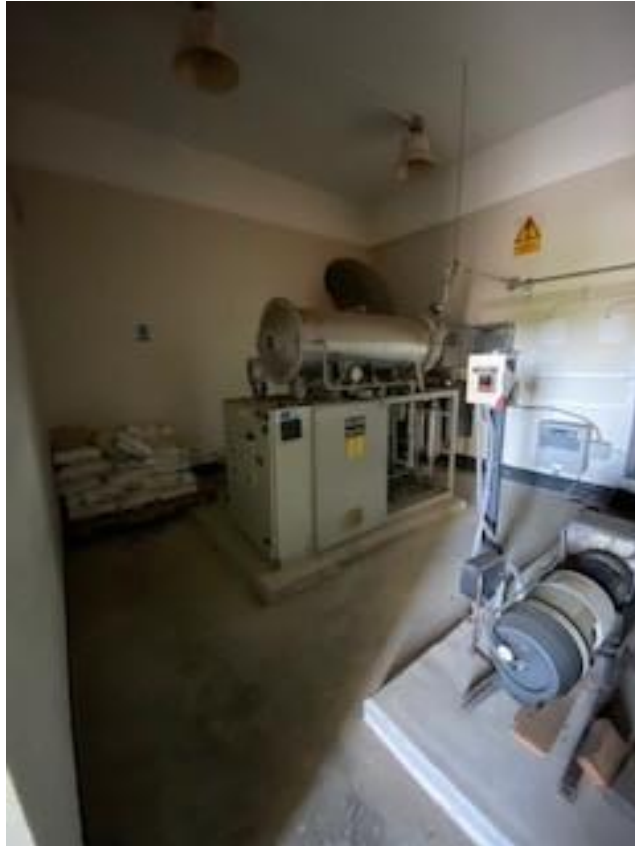
Figure Y. Ozone Disinfection System (abandoned / not in operation)
