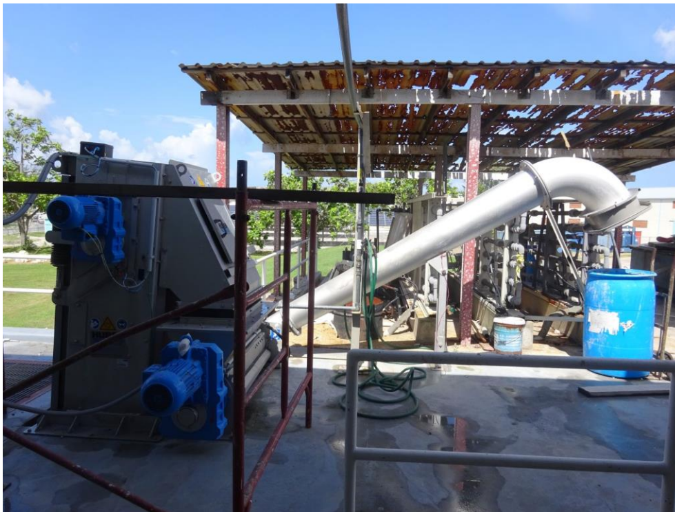
Figure DD. Inlet Course Screen System (not installed)
