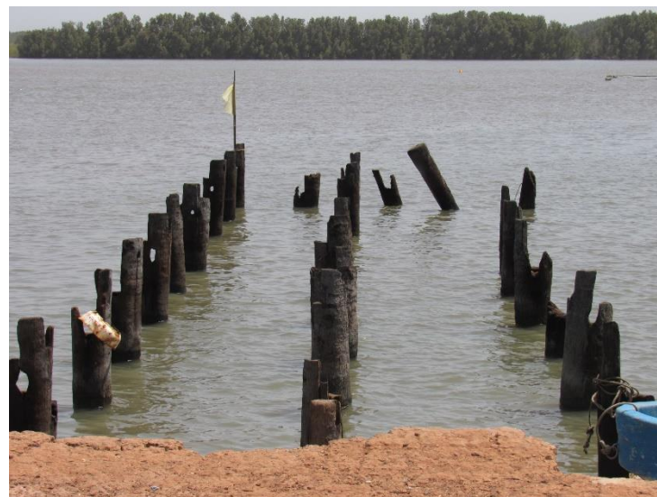
Figure 21 –View of level of river bank ( left ) – Existing jetty piles removed ( right ) and replaced with floating pontoon
