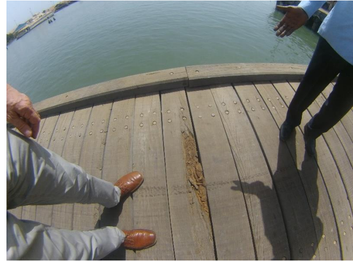
Figure 3 –Timber deck on existing jetty requiring maintenance
