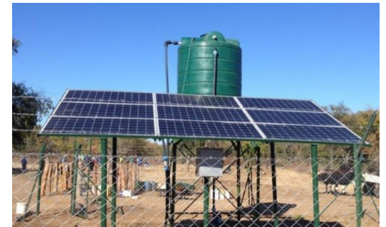
Solar powered seawater borehole for fish rinsing
