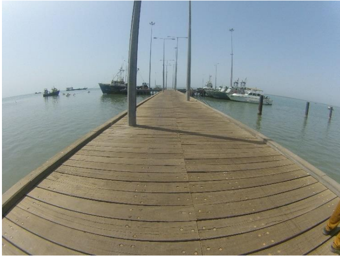
Figure 3 –Timber deck on existing jetty requiring maintenance
