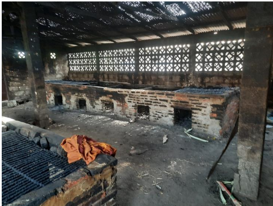
Figure: Fish smoking house with dilapidated roof at Kartong river landing site
