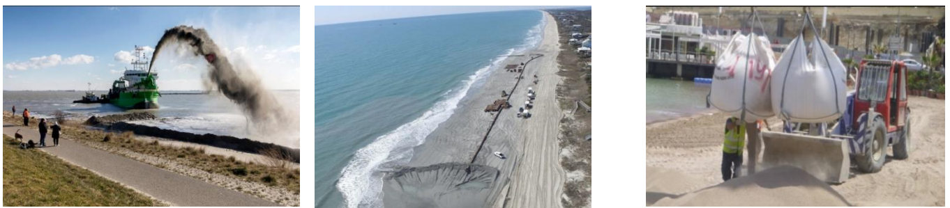
Figure 6 Sand replenishment on a large beach (by pumping) and a small beach (by dumping)
