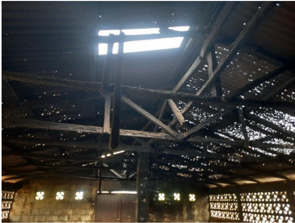
Figure: Poor roof and rainwater inlet into the smoking house
