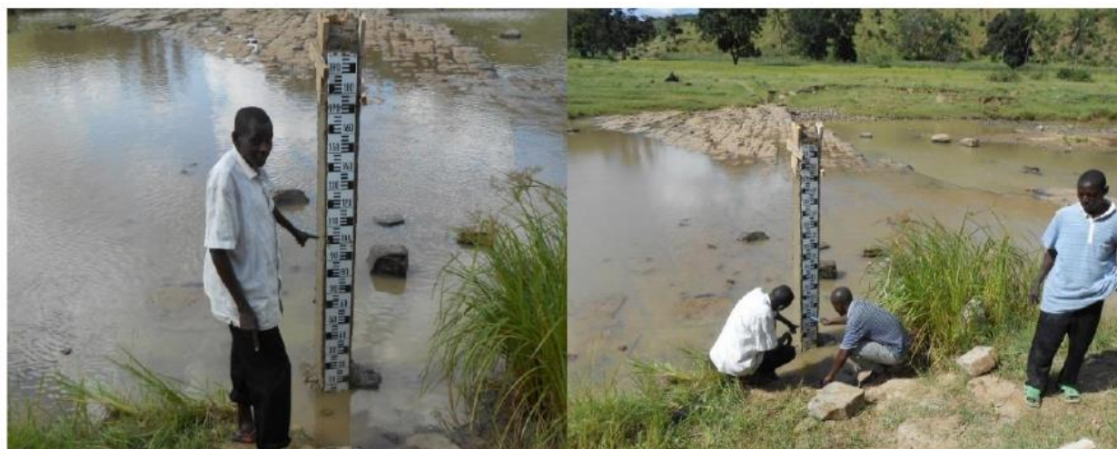
Figure 52: Concrete Post Installed at Mwache 3 MB02 and Gauge Reader in the Athi Catchment Area
