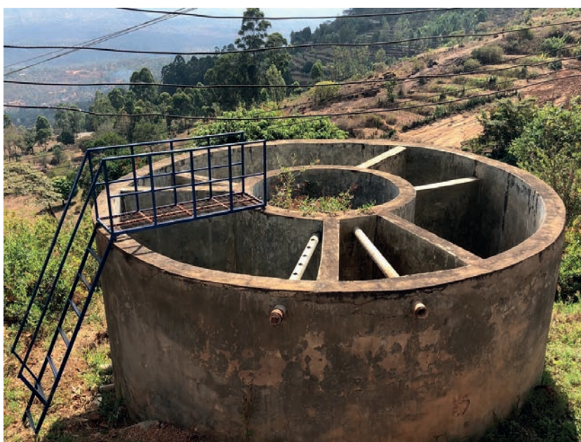
Figure 85: A leaking CFU in Muooni water pan proposed for rehabilitation
