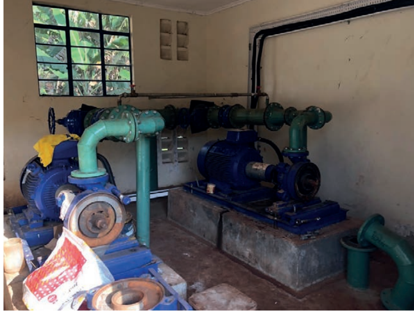
Figure 71: Pumping solution that rely mainly on grid power hence expensive to maintain
