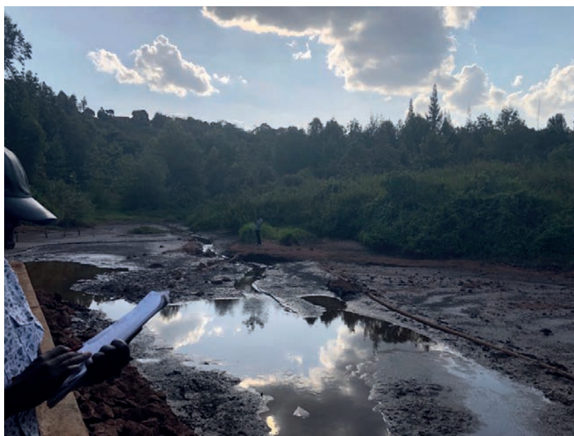
Figure 70: Kikuyu spring sump that requires rehabilitation
