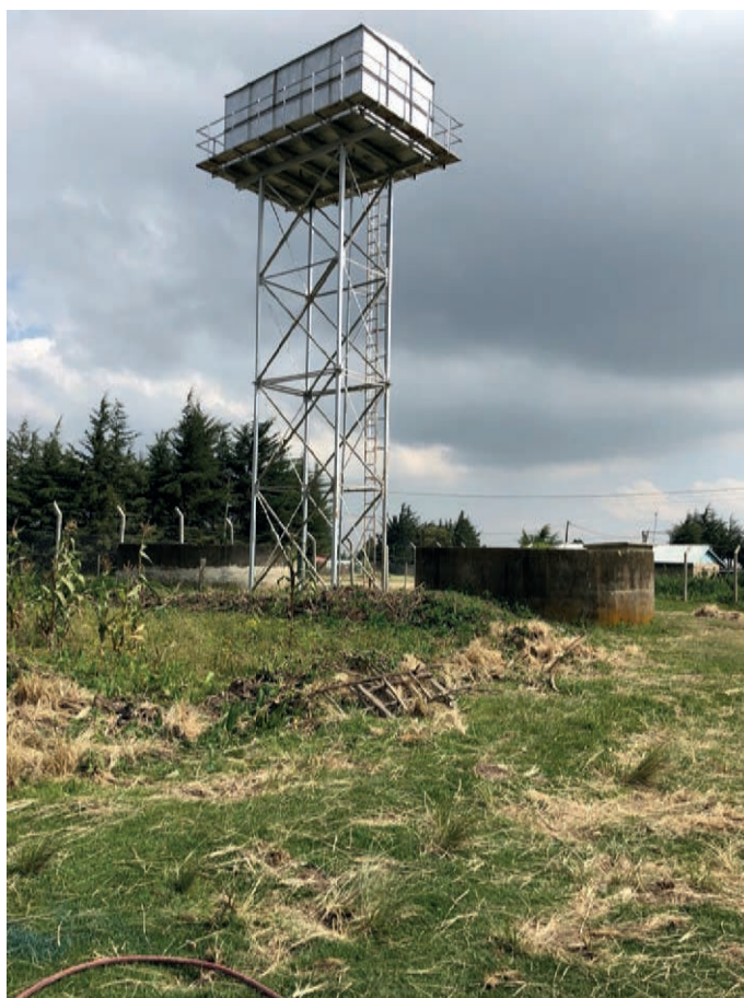
Figure 28: Metallic elevated tank in Koinange borehole
