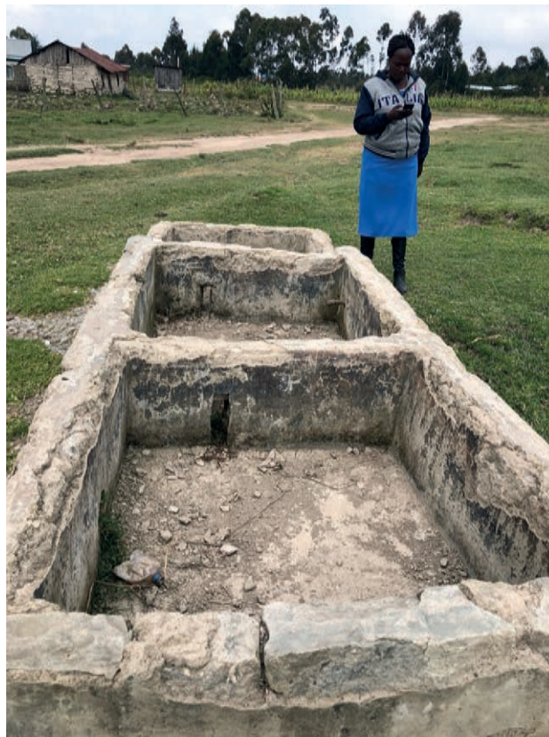
Figure 25: A cattle trough that is leaking and in need of rehabilitation
