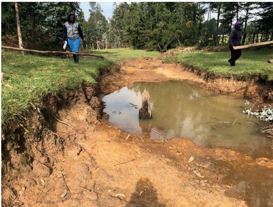
Figure 32: An eroded spillway in Wachira Waheni water pan
