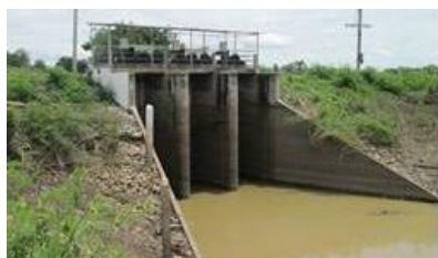
Existing Wang Khon Culvert 3 @ 2.90 x 3.00 m (looking upstream)
