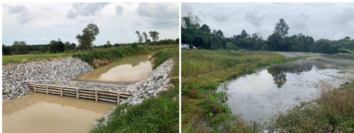
Figure 5 Micro dam in Haui Sai Bat (left) and sediment trap wetland in Thai Di (right) designed and constructed by DWR
