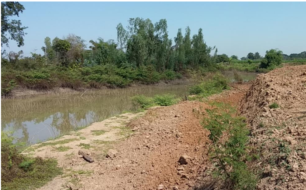
Figure 11: Cross-section with an unvegetated berm (foreground)
