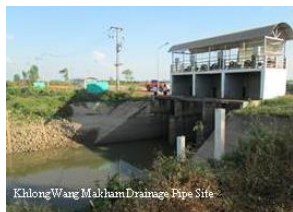
Existing Wang Makham Culvert 3 @ 3.00 x 3.00 m (looking upstream)
