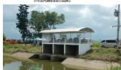
Existing Wang Won Culvert 3 @ 2.90 x 3.00 m (looking upstream)
