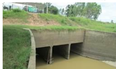
Existing Wang Khon Culvert 3 @ 2.90 x 3.00 m (looking downstream)
