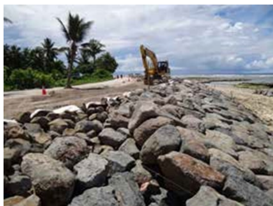
Figure 31: (Annex) Rock revetment at South Tarawa, Kiribati
