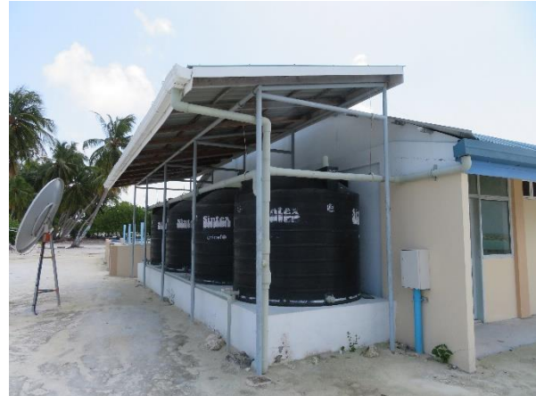
Figure 2.4.7 Rain Water Storage Tank in Maabaidhoo
