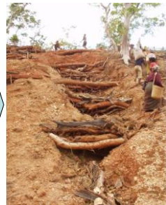
Erosion control with wattles
