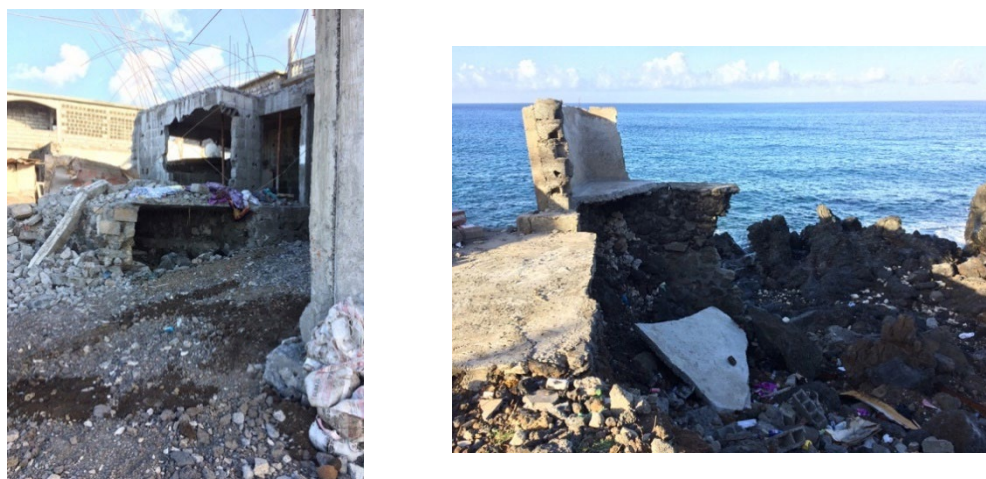
Figure 61 Damaged coastal defence leaving coastal buildings close to sea unprotected
