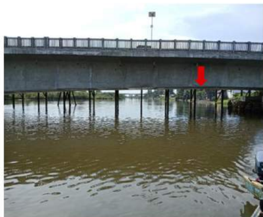
Figure 3.10: Vertical clearance height Bong Mine Road bridge. Left panel: photo of bridge with red arrow indicating which point at the bridge bottom has been used. Note: the steel pillars in the back correspond to the Bong Mine Pipe Bridge which is treated in the next section. Right panel: schematic of determined distances. Total vertical clearance height: 271.5cm
