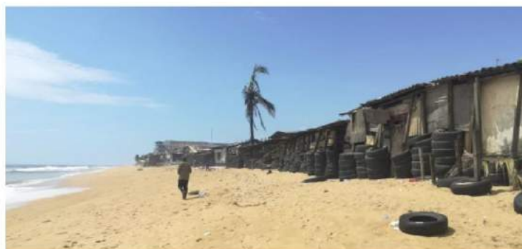
Figure 4.6: Car tires on the beach to protect houses
