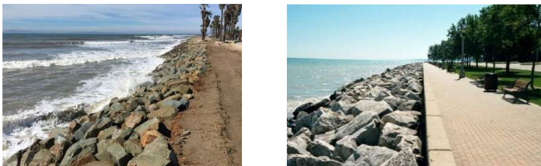
Figure 6-13: Examples of rip-rap revetments
