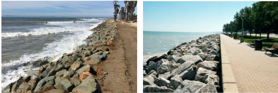
Figure 2-3 Examples of rip-rap revetment walls
