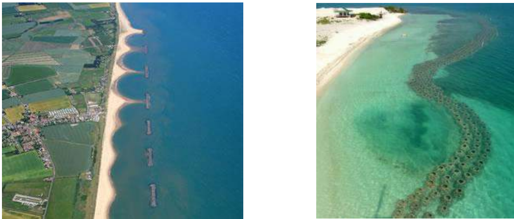
Figure 6-12: Left series of emerged detached breakwaters, Right a continuous reef breakwater
