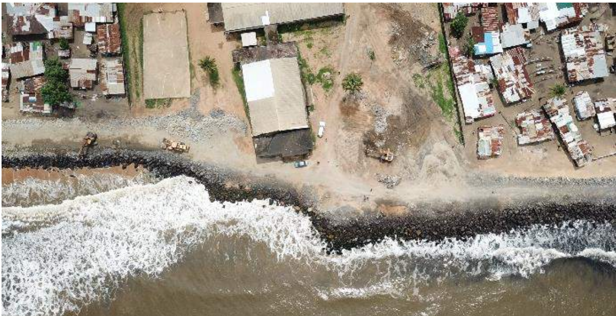
Figure 7-2: School at the shoreline, being protected by a rip-rap revetment (Oct 2018)
