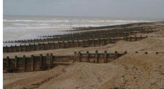
Figure 6-9: Groyne structures (Left long impermeable groyne, Right series of short permeable groynes)
