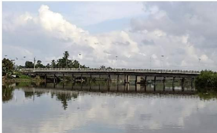
Figure 3.11: Bong Mine Pipe bridge. This bridge is the steel construction in front of the concrete structure which is the Bong Mine Road bridge.
