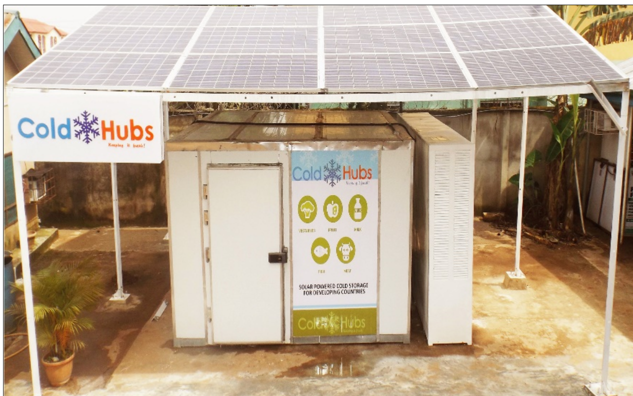
Figure 22. ColdHubs – walk-in solar-powered cold storage units – in rural Nigeria 110 .
