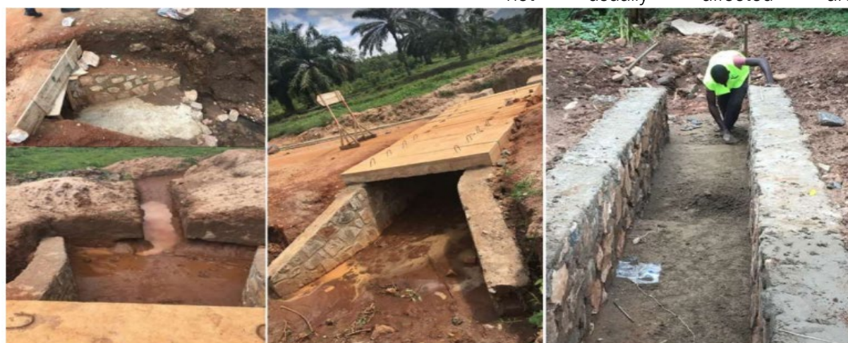
Figure 1 : The provision for culverts to drain storm water runoff has been found to be inadequate in the slopes and PNSADR-IM has to extend these, making is more costly.
