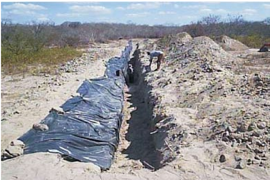
Photo L- Placement of canvas for the construction of an underground dam 315 .
