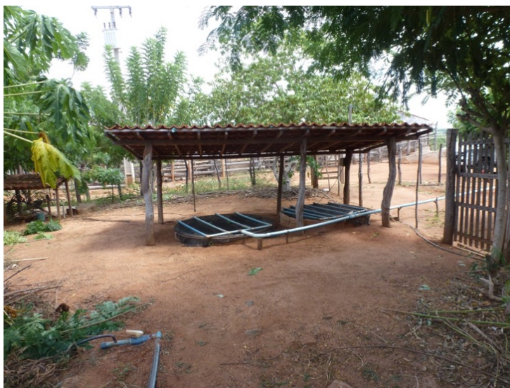
Figure 45 Biological filters from Family Biowater System, with plumbing bringing gray water from the house. In this case, the graywater 'production' is significant, justifying the double filter 184
