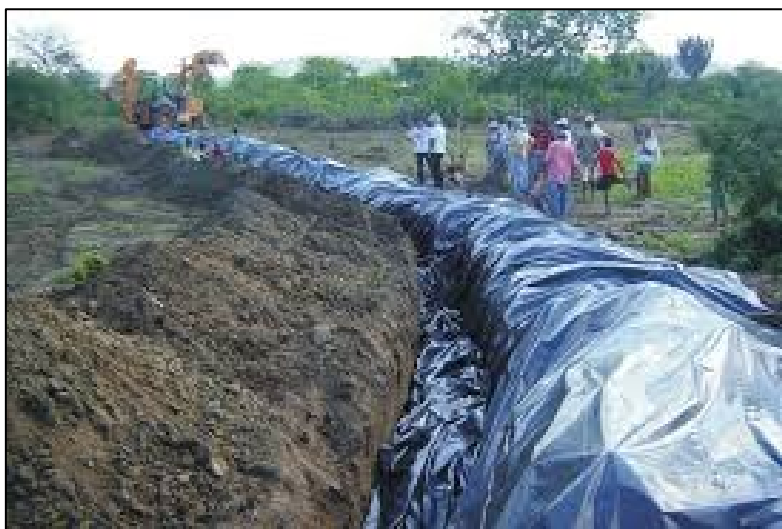
Figure 43 Waterproof tarpaulin installation of an underground dam under construction 176
