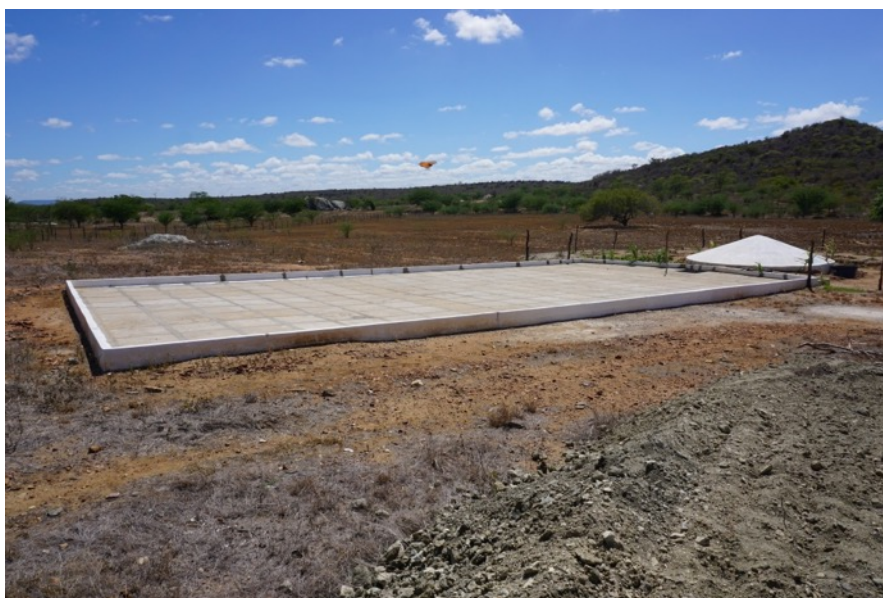
Figure 41 Rainwater harvesting and storage boardwalk with its 52,000-liter cistern. 168
