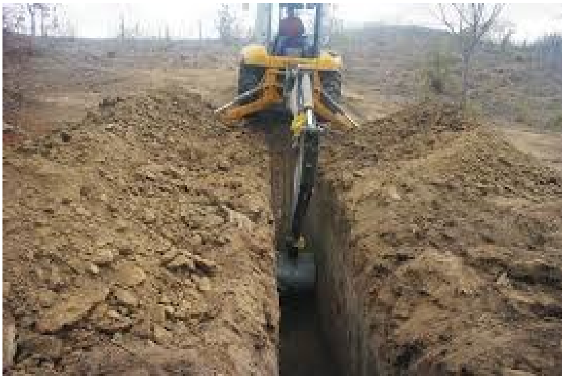
Photo K- Tractor with mechanical shovel dug into an underground dam (BS) 314
