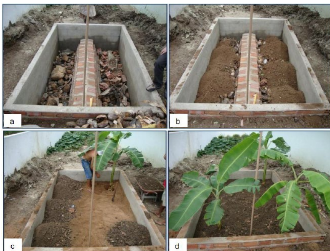
Figure 47 Step by step construction of green septic modules in the Paus Broncos community, Settlement May 25th, Ceará. 199
