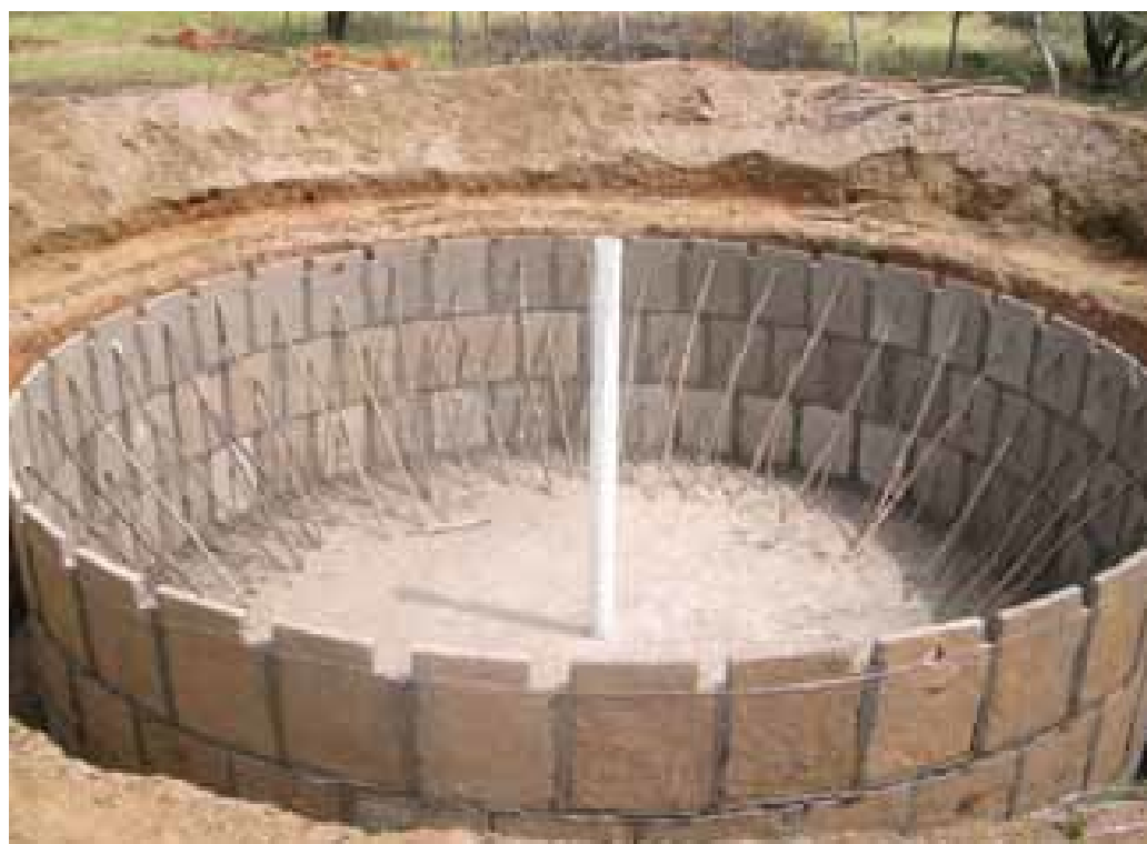
Photo H – 52 thousand litre cistern in construction 311
