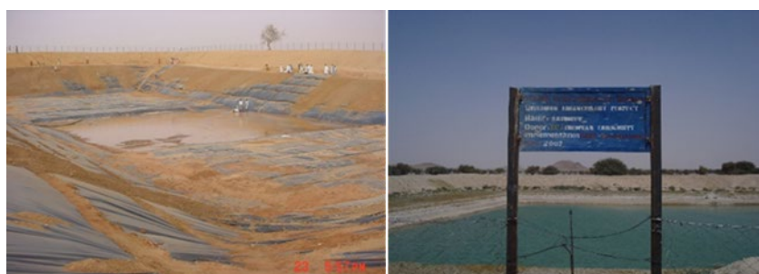
Figure 2-3: Pictures of a hafir under construction (left) and an operation hafir (right)
