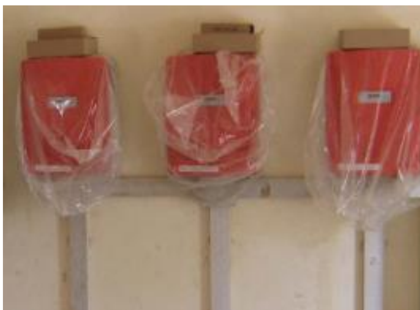
Photo 3: Example of single-phase inverters
