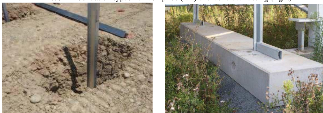
Photo 2: Foundation types - driven piles (left) and concrete footing (right)
