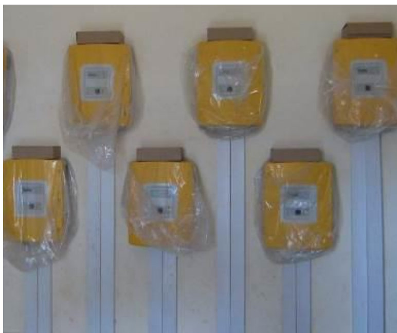
Photo 2: Example of Sunny Island 48VDC/230VAC photovoltaic inverters
