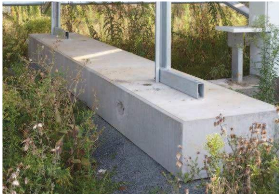
Photo 8: Foundation types - driven piles (left) and concrete footing (right)
