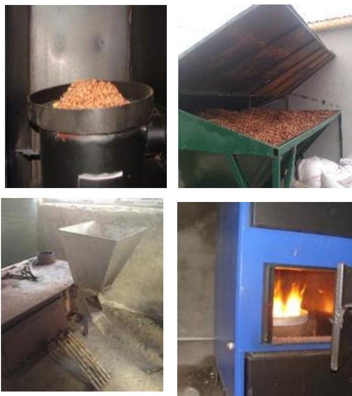
Figure 70: Use of hazelnut residues for heat supply
