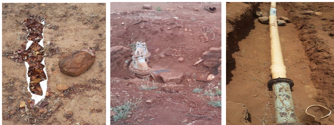
Figure 16: Broken pipes
