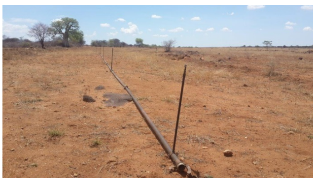
Figure 20: Out of service sprinkler system at Mzingwane scheme
