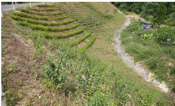
Bio-engineering solution for protection of slope and drainage system in Thai Nguyen (ICEM)
