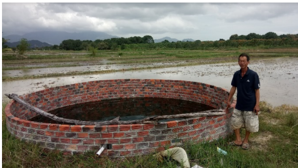
Figure 64: A typical pond to collect and store shallow ground water for perennial crops in Cam Hiep Nam communes in Cam Lam District, Khanh Hoa
