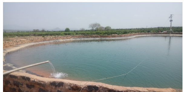
Figure 70: A model of pumping well and storage pond for large scale farming (50ha) in Bac Binh, Binh Thuan
