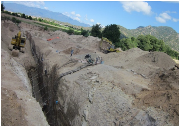
Figure 67: Building of underground weir for ground water exploration in Thuan Bac, Ninh Thuan
