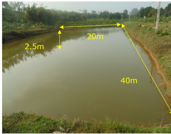
Figure 39: Simple design of a pond for 0.66 ha irrigation of non-rice crop
