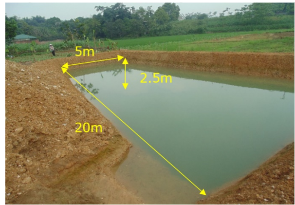
Figure 40: Simple design of a pond for 0.13 ha irrigation of non-rice crop
