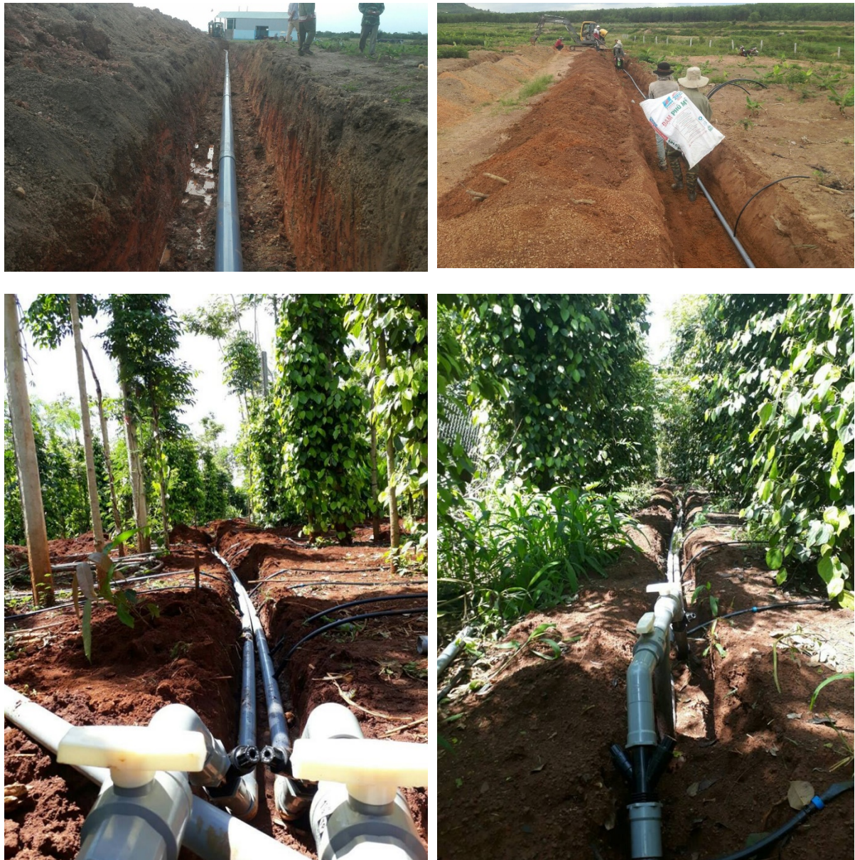
Figure 51: Buried pipes for HEI application in Central Highlands (Netafim Dak Lak)
