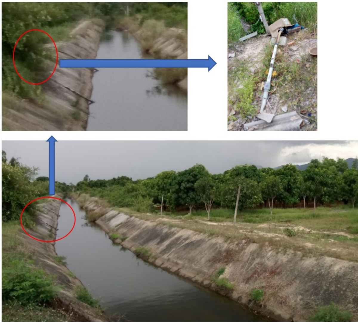
Figure 20: The exist private pumping systems from opened canal in subproject area in Khanh Hoa: the pipe from canal and the electrical pump in canal-bank
