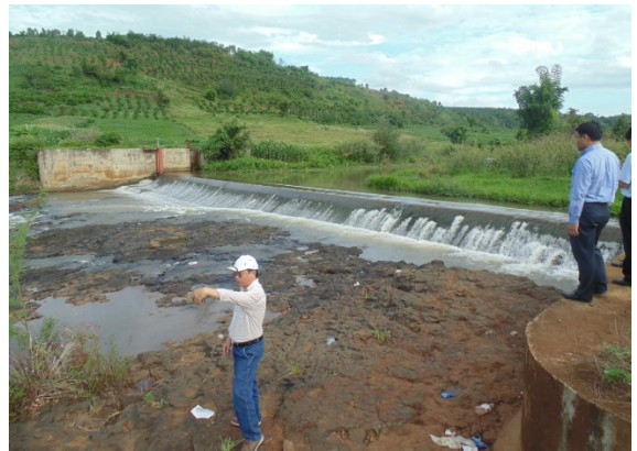
Figure 63: A checked dam for irrigation in Cu Jut district
