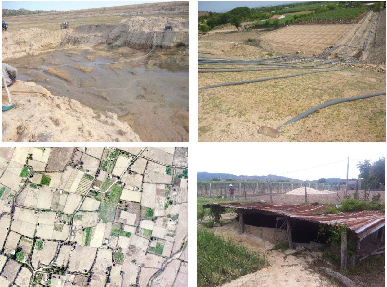
Figure 23: Digging within Ong Kinh reservoir to get water for irrigation and private pipeline from the pumps to irrigation area (above)). Excavation wells for groundwater extraction in field plots (black dots) and anti-evaporation shield design for wells in Nhon Hai (below)
