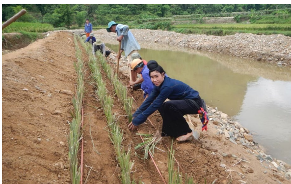
Bio-engineering solution for bank erosion protection in Bac Can province (ICEM)
