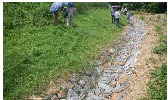
Bio-engineering solution for protection of slope and drainage system in Thai Nguyen (ICEM)
