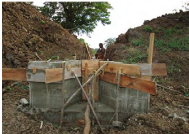
Figure 79: Structural measures in tank rehabilitation
