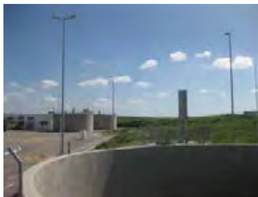
Figure 12-32: Flare near to the gas holder. Sludge silos in the background
