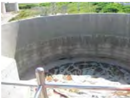
Figure 12-31: Future gas holder; storage Facility for biogas
