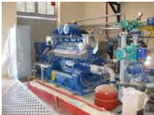
Figure 12-22: Biogas-engine
