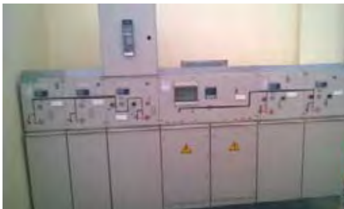
Figure 12-26: Ring-Main-Feeder switchgear
