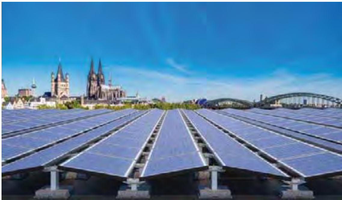
Figure 5-2: East-West orientation on a roof-top, press photo by manufacturer Renusol
