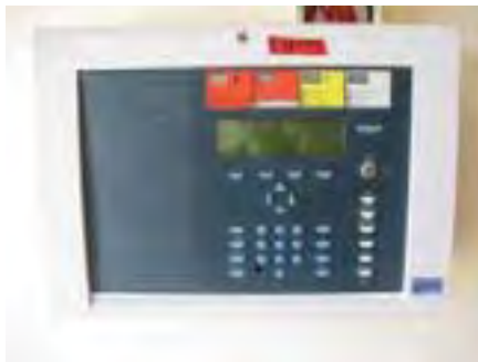
Figure 12-29: Fire detection unit
