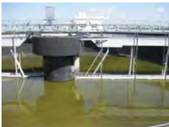
Figure 12-41: Final clarifier (1 of 3)
