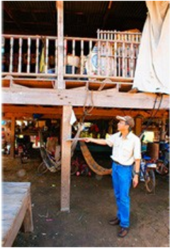
Normal flood level
