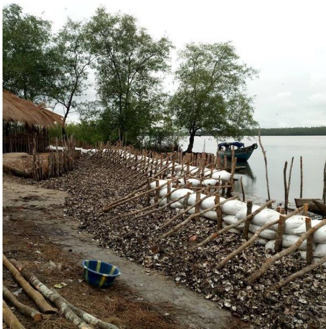
Figure 86. Example of community micro-scale artificial coastal protection measure built with support of the WA BiCC project using local materials of wood, oyster shells and sand bags 426
