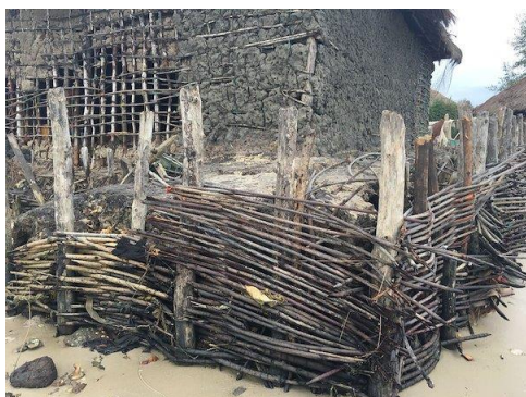
Figure 84. An example of woven wooden fences erected by communities themselves in an effort to combat coastal erosion and reduce flooding. Source: WA BiCC 424
